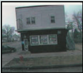
Family Store with living quarters above
